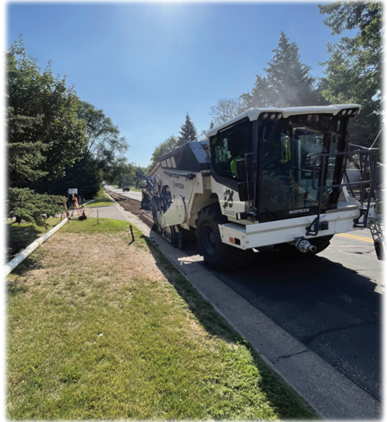
Reclamation on Cope Avenue (2022)
