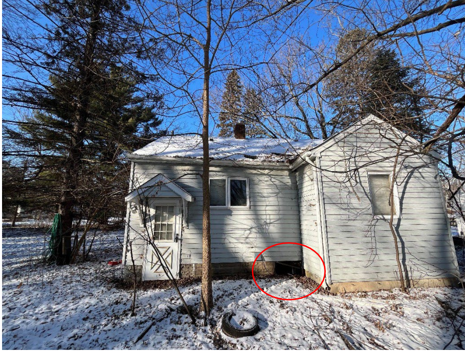
Photo 18 – Opening in the foundation wall that allowed photos
