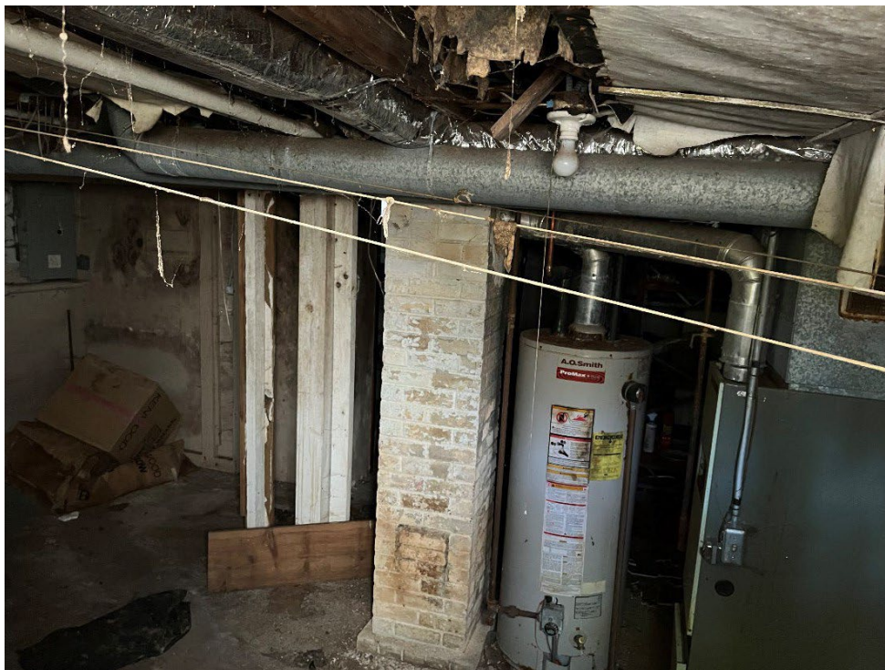
Photo 19 – Basement area through the foundation wall opening
