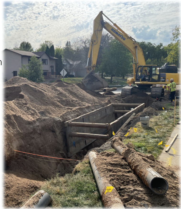
Water main replacement Cope Avenue (2022)
