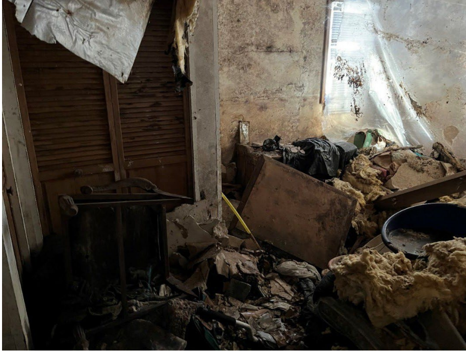
Photo 12 – Contents of the bedroom
